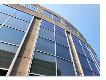
Over the decades, the building's exterior curtainwall experienced significant deterioration and was leaking air into the building. The glass curtainwall had a number of failed insulating units, and the original manufacturer no longer made the system used on the building. Therefore, the project and ownership teams needed to identify a custom solution that would meet the performance requirements for the building's restoration while staying within the budget established by the state of Wisconsin.
