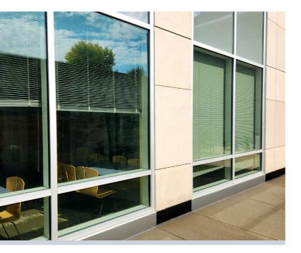
The project team needed to work within the parameters of a building with a completely sealed envelope from the exterior with no weeps to drain water. Therefore, they needed to work within the already established barrier system while upgrading the necessary components.
